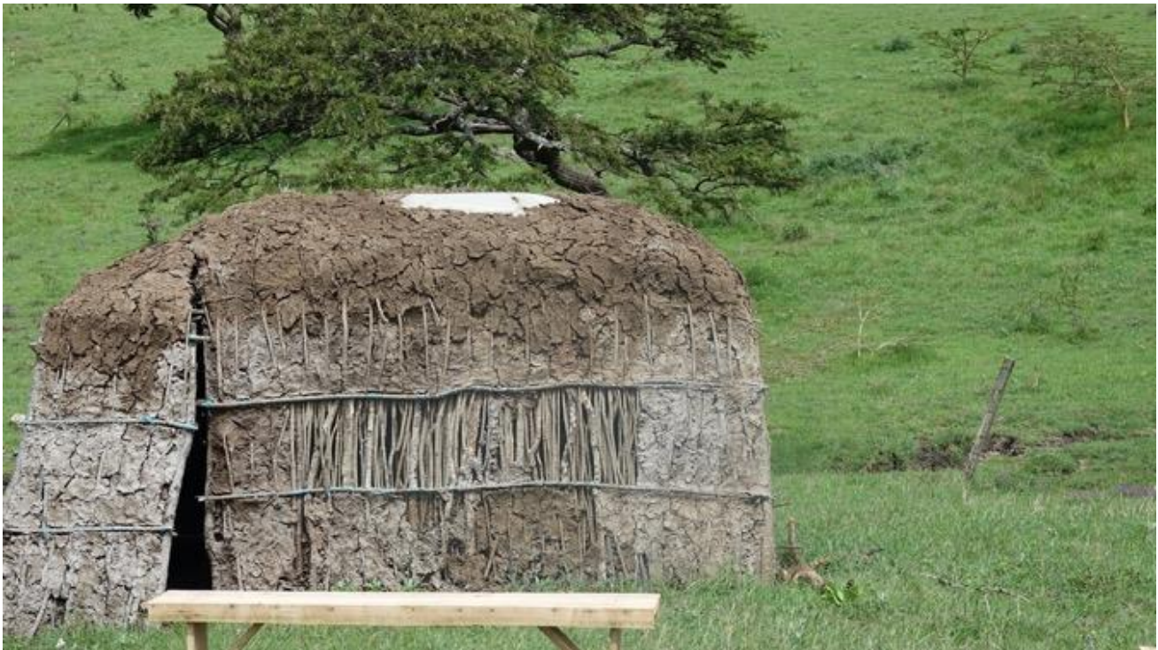
This manyatta, is where we made our bracelets. It's the traditional home of Maasai. The manyatta is built by women, made from cow dung, urine, and grass and it's made to be impermanent. These huts take a year to build. Female family and friends are recruited to help because building huts and caring for family are the domain of Maasai women.
